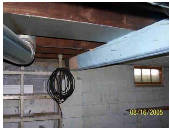
UNDER FLOOR SPACE (5)
